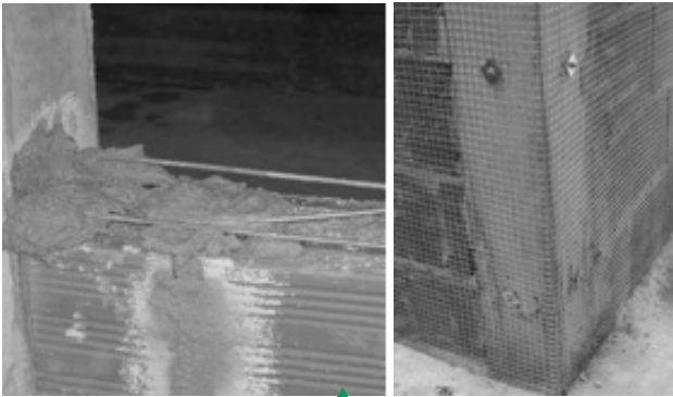
Bed joint reinforcement | Reinforced plaster
