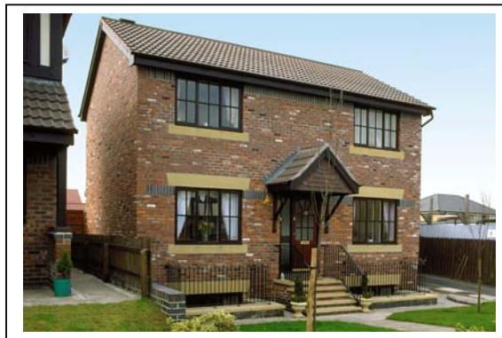
Figure 5d: A brick and block house with a basement, Manchester, UK. (Courtesy of the Basement Development Group)
