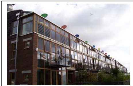
Figure 1a Heavyweight construction coupled with a design that incorporates sun spaces makes the most of solar gain and thermal mass. at BedZED, a zero energy development in London. (Photo taken during study tour at BedZED)
