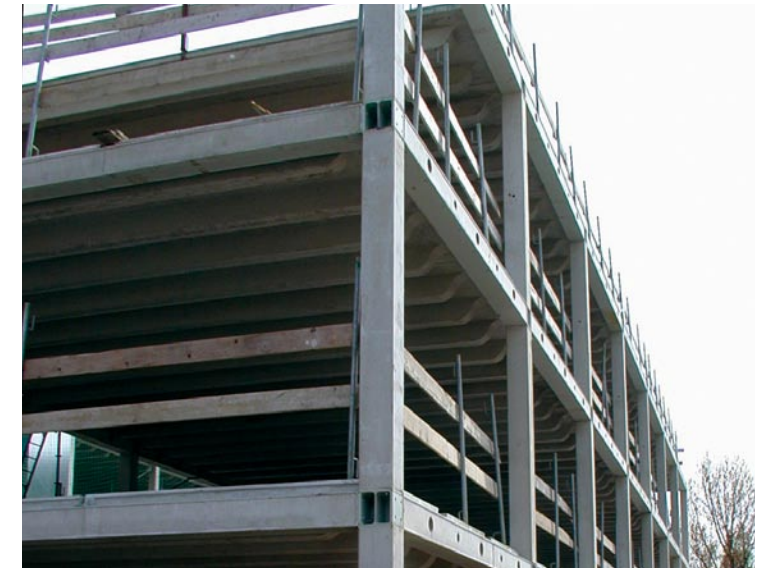
A building's demountable skeleton in the Netherlands. Courtesy of BFBN.
