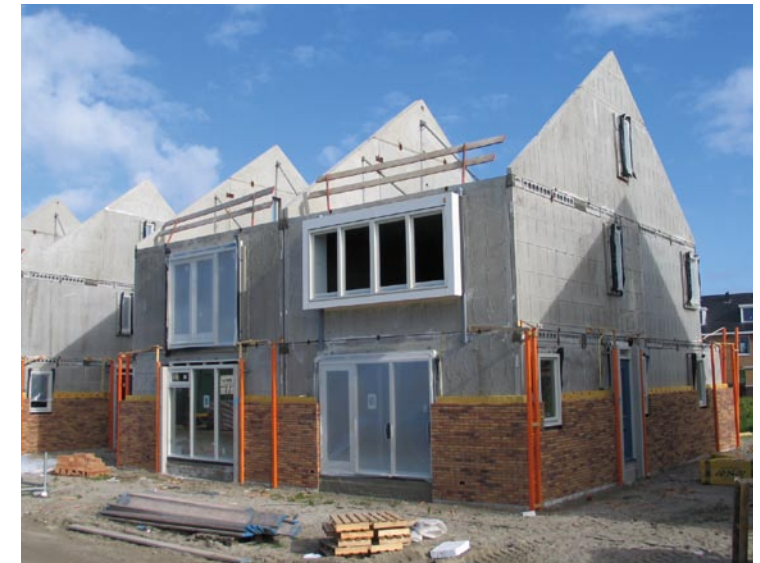
Lightweight concrete blocks are widely used in foundations and external walls for small houses because they are easy to lie and easy to work with. Courtesy of BFBN.
