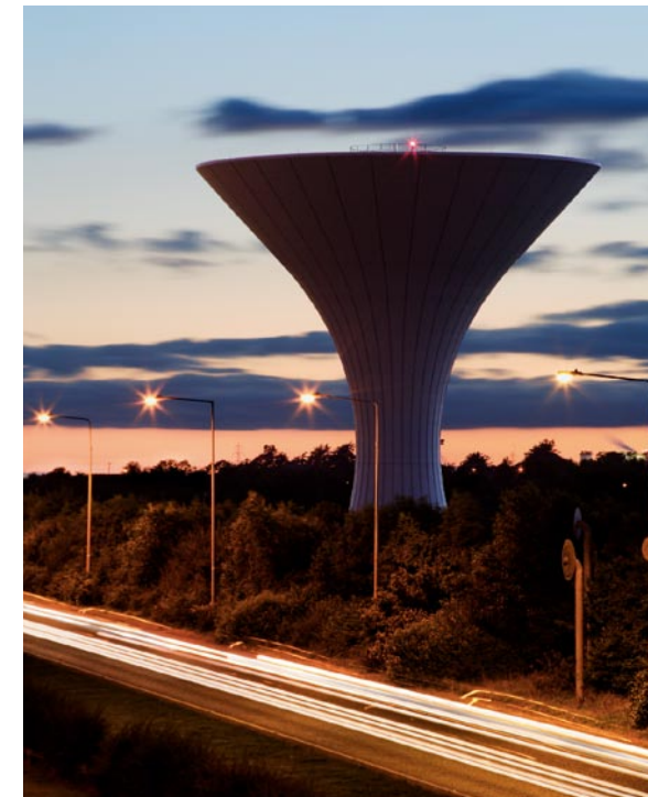
Example of the Sillogue Water Tower. Courtesy of P.H.Mc Carthy Engineers, Dublin, Ireland.
