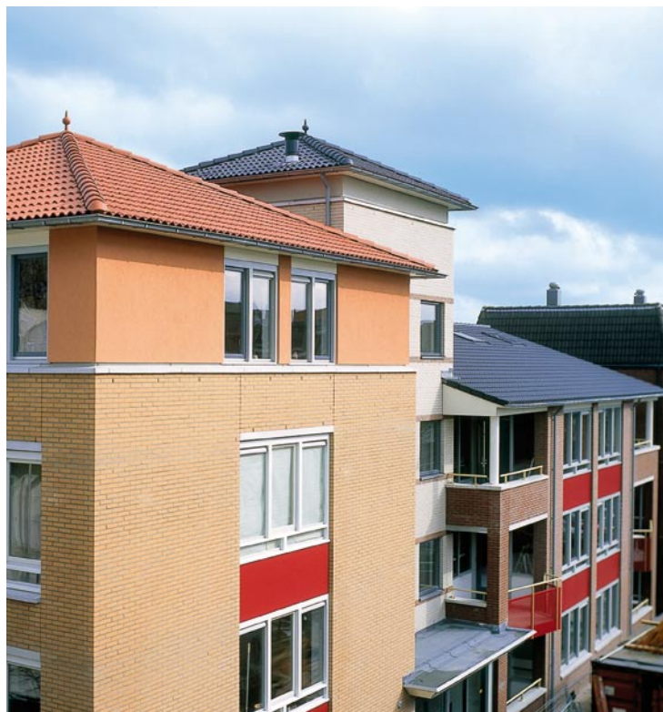
Dutch buildings made of precast concrete units. The concrete roof tiles used for the roof finish ensure a long service life for the building. Courtesy of BFBN.
