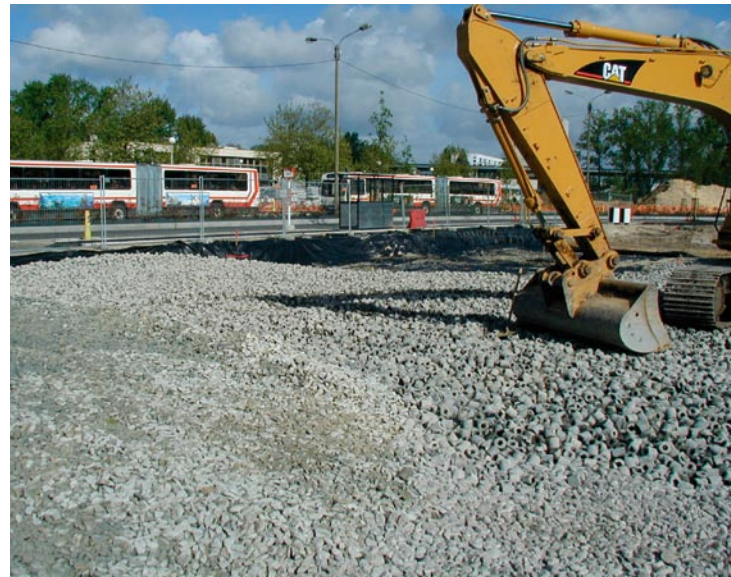
Recovered waste material and crushed waste concrete can be used in road construction. Credits: Photothèque CERIB.
