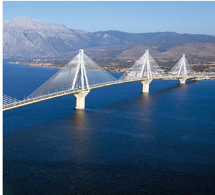
The 'Rion-Antirion' suspension bridge in Greece is a structure that calls for a long service life. The bridge is 3km long and the centre span is 560m long. Courtesy of FIB.
